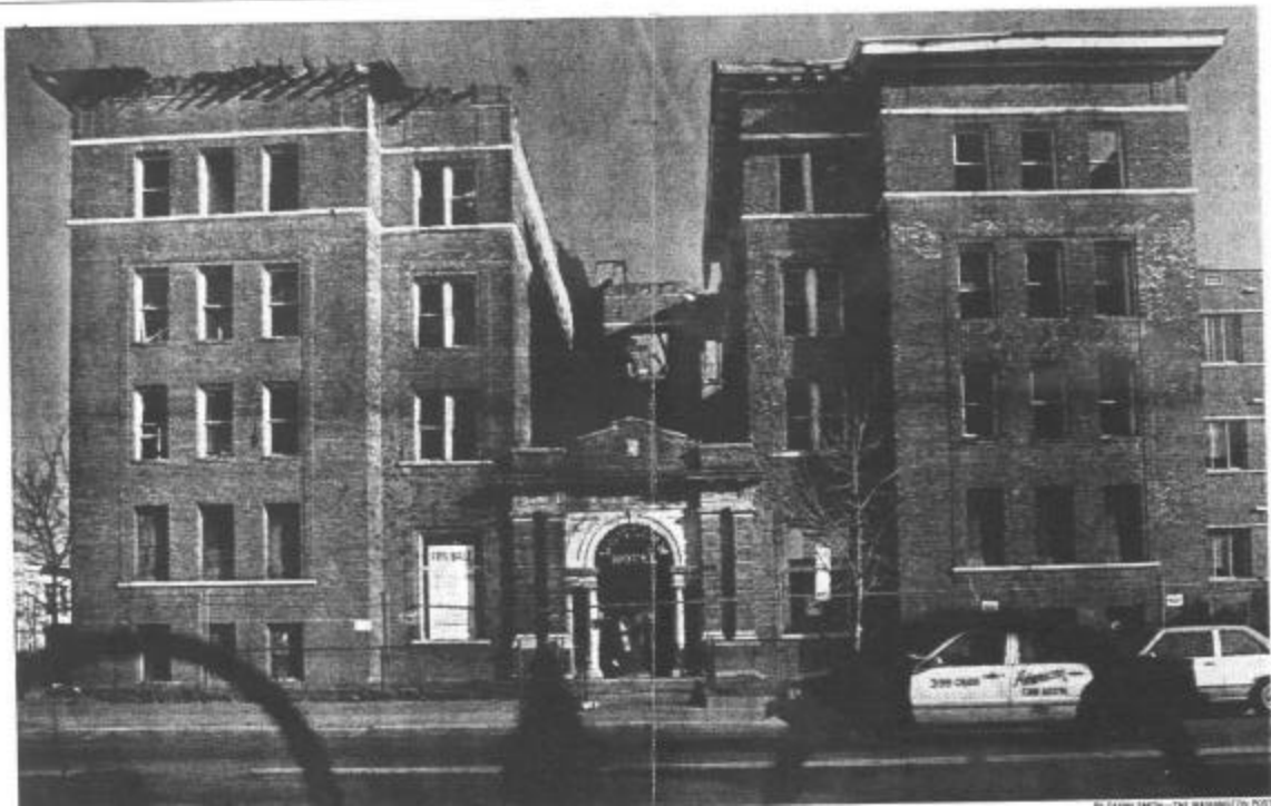
Figure-1, The Whitelaw Hotel prior to renovation, 1979. Washington Post, 02 January 1992.
