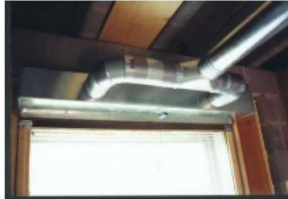
Figure 4.17 Air outlet slot connects to ducts
